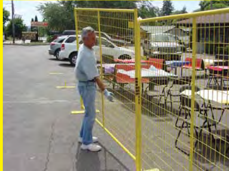
Simply place panel on top of bases and the fence begins to take shape
