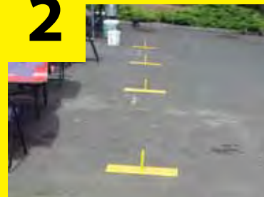
Place bases approximately 7.5 feet apart around perimeter of job site.
