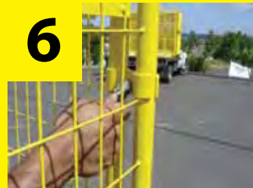
Connect panels to each other using the panel clamps.
