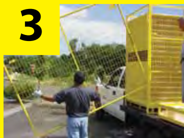
Remove a panel from the pallet.
